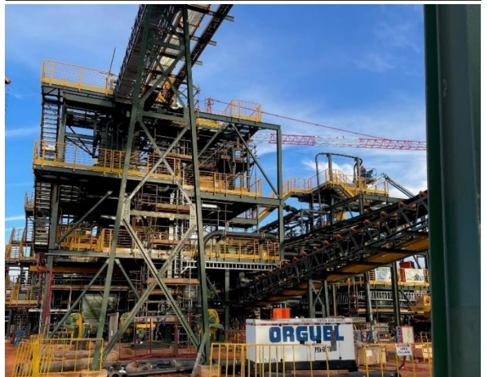
Figure 4: Dense Media Separation plant ~80% complete
