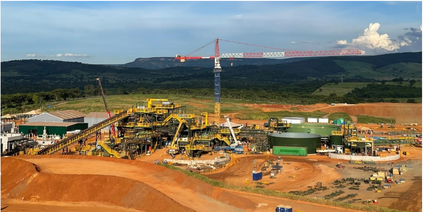
Figure 5: Bird's-eye view of Dense Media Separation plant construction
